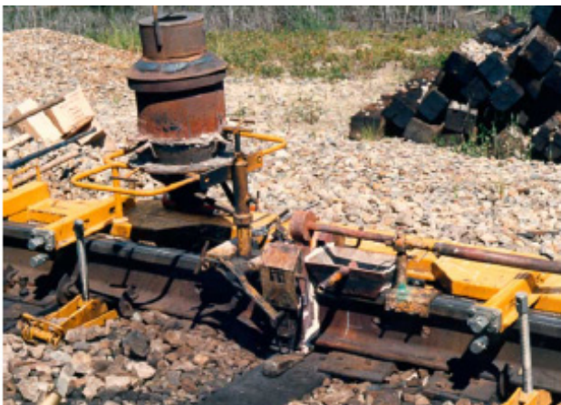
Fig. 1. Aluminothermic welding (with melting) [10]
