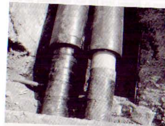
Figure 1b: Details from the building site
