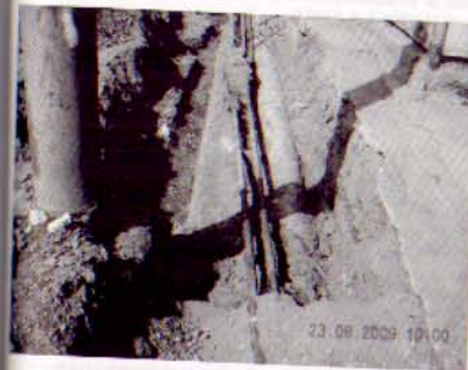
Figure 1a: Details from the building site
