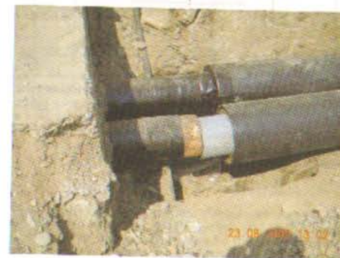
Figure 3: It is important to make pipes coaxial
