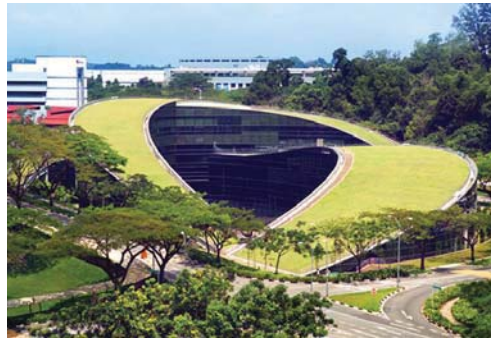
Figure 6 Curved green roof
